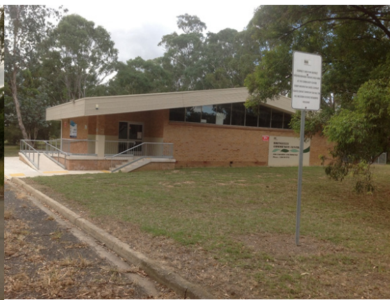
Figure 7-46 View north of Bringelly Community Centre from Greendale Road
